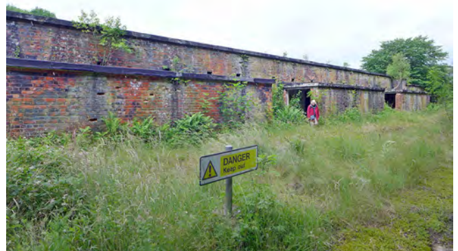
Changing rooms in the 'Danger Area'. The 'Danger Area' which was isolated from the rest of the site is where the manufactured munitions were charged with fuses and detonators. The road surface changed from concrete to Colas in this area. This was to reduce the risk of a spark from something being dropped onto the floor igniting one of the weapons being filled
